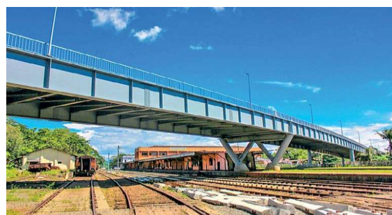
Recently completed Polgahawela Flyover under Spanish assistance
