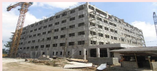
Construction works of Maternity Hospital, Galle
