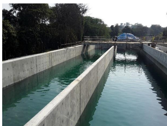
Construction of Oxidation Ditches
