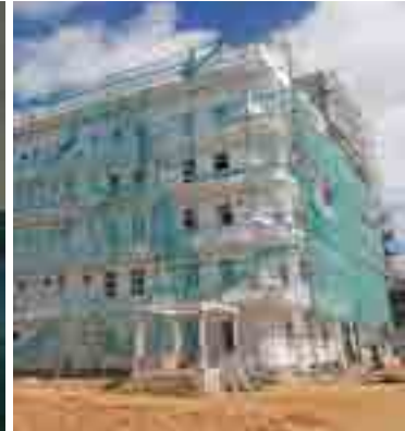
Construction of DGM(NCP) Office in Anuradhapura
