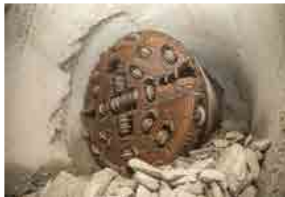
Main Tunnel Breakthrough
