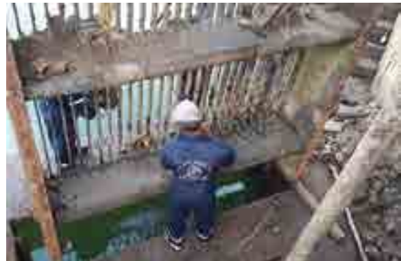
Repairing of trash rack
