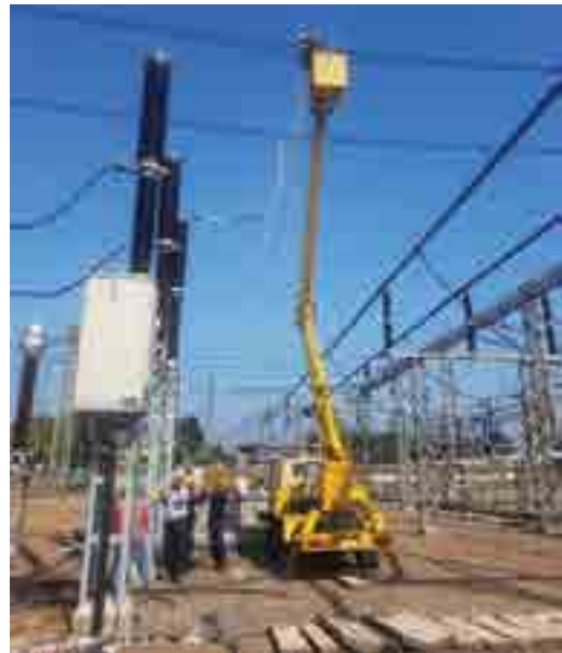
Figure Tr.12: Down dropper replacement work
