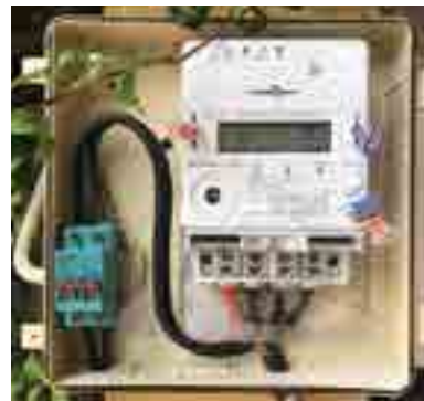
Smart meter installation under pilot project
