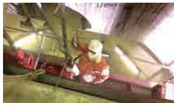
Sand Blasting and Painting of Intake Gate, Draft Tube Gates and Surge Chamber Gate at Kotmale Power Plant.
