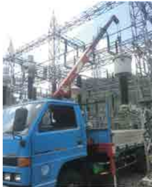
Figure Tr.10: Replacing 132 kV CTs at Ukuwela GS
