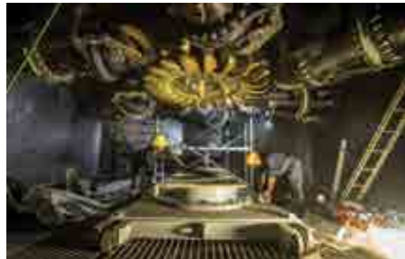
Installation of Turbine (Unit1)
