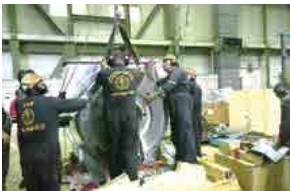
Installing the new TCA66 Turbocharger
