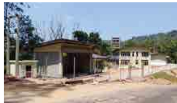
Construction work of the new Employers Office building
