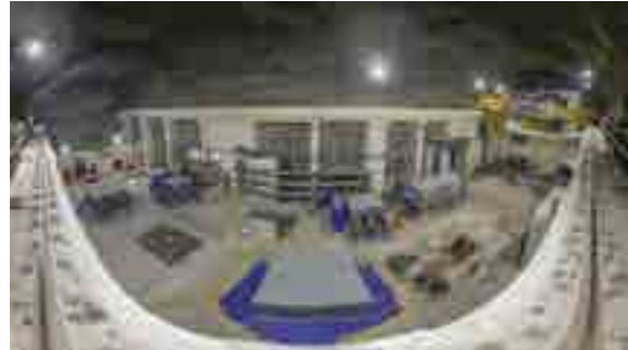
Present View of Power House Machine Hall Floor
