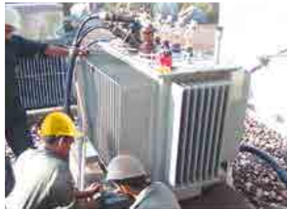
Installation of New Auxiliary Transformer for Kotmale Switchyard
