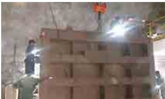
Sand Blasting and Painting of Intake Gate, Draft Tube Gates and Surge Chamber Gate at Kotmale Power Plant.
