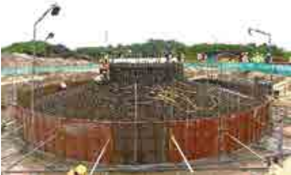
Site works in progress- MWPP
