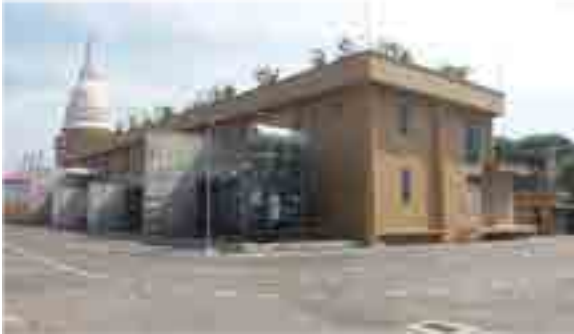
Colombo L Grid Substation
