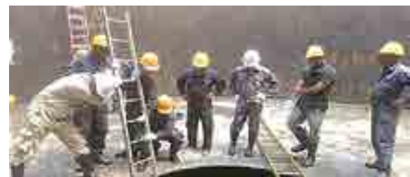
Accessing to Tunnel
