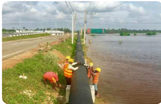
Pipe laying along A9 Road
