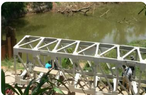
Steel Struss Work at Bridge no. 33/3
