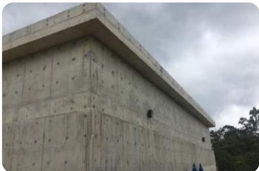
Jayasinghagama 800m 3 Tank after completion
