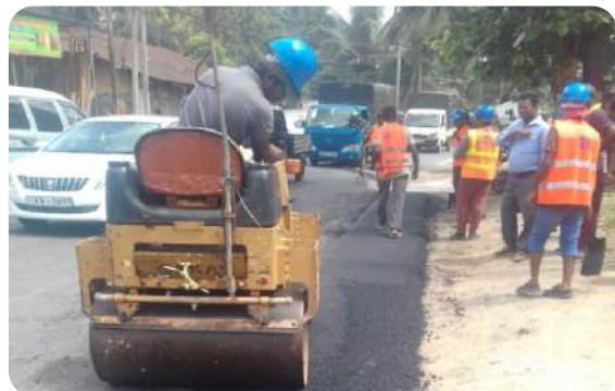
Permanent road reinstatement after the pipe laying
