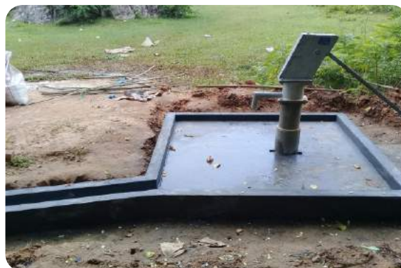
Hand Pump Well Construction - Nuwaraeliya
