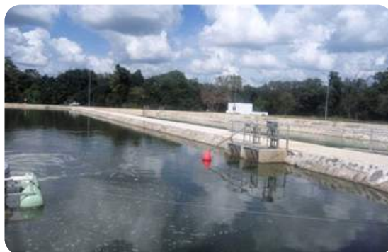
Completed Aerated Lagoon
