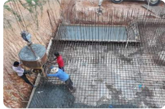
Concreting the Base of Ground Reservoir in Weligama WSP
