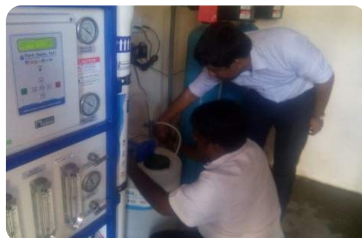
Installation of RO Plant
