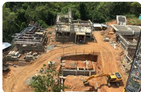
Construction of Water Treatment Plant at Sulugune
