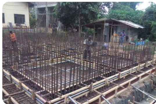
Reinforcing of Sedimentation Tank
