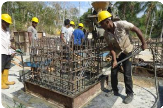
Chamber concreting
