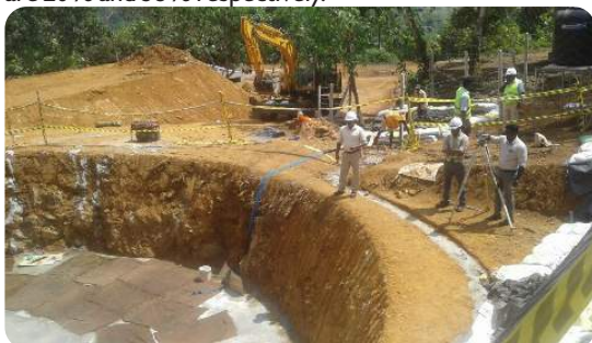
Foundation Excavation Neboda Water Tower
