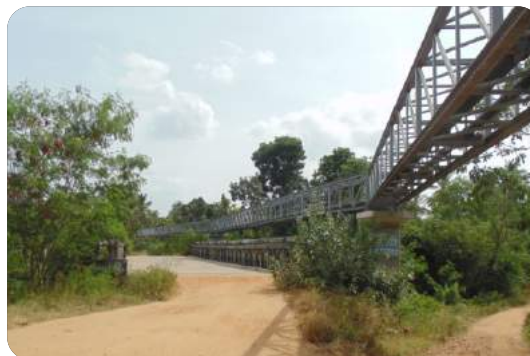
Completion of Pipe Bridge
