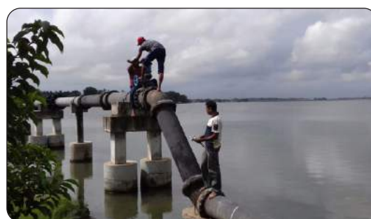
Air valve servicing in Transmission main at Batticaloa
