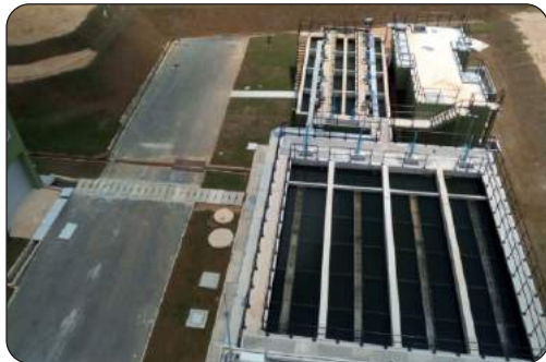
Puttalam Water Treatment Plant
