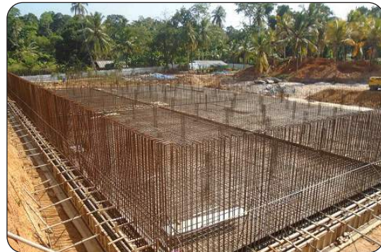
Water Treatment Plant site
