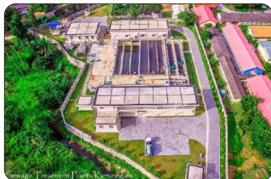
Sewerage Treatment Plant
