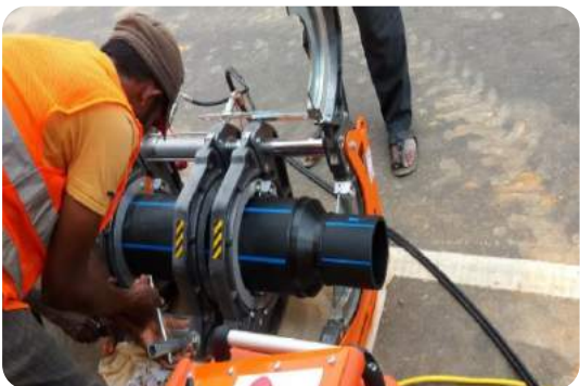
Pipe Laying Work of Distribution System
