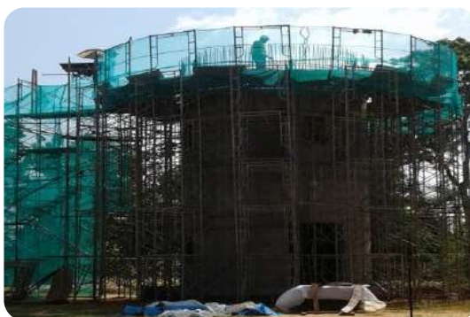
Kotawehera Water Tower
