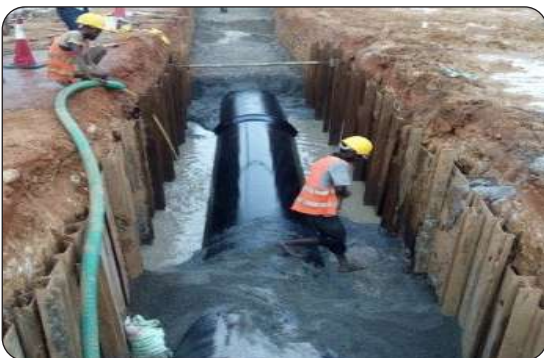
Orugodawatta Pipe Laying
