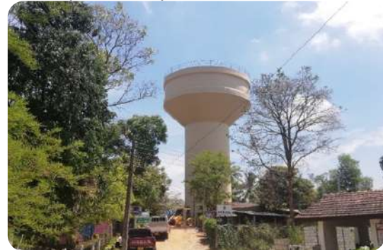
1,000 cu.m capacity water tower at Mawathagama
