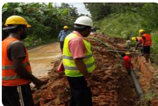
While completing a Type "B" Culvert Crossing at Dikkumbura WSP
