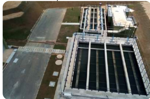
Puttalam Water Treatment Plant
