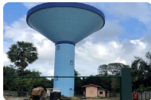
Serunuwara Tower Construction
