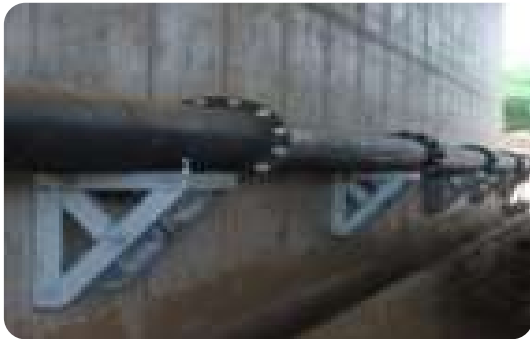
Highway underpass pipe laying at Bandagiriya
