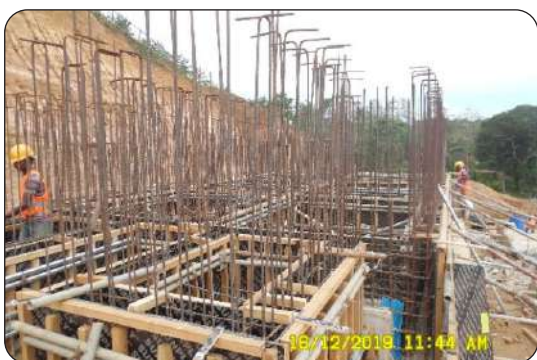
Coagulation & flocculation tanks
