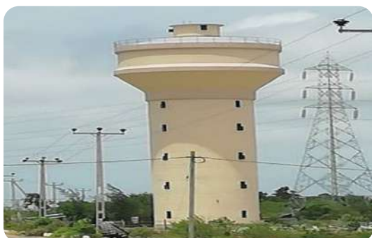
Completed Water Towers
