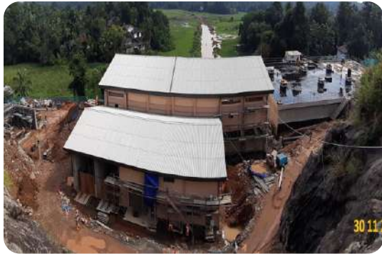
WTP Construction progress
