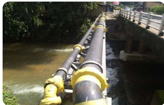
Pipe laying across the Bridge No. 53/3, Avissawella
