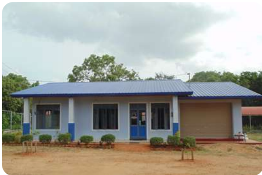
Office Building at New Town tower Premises
