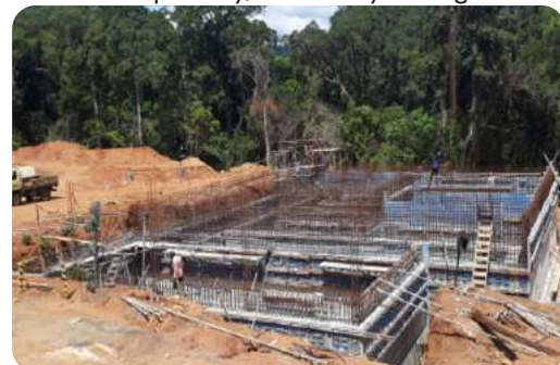
Construction of Clear Water Reservoir at WTP
