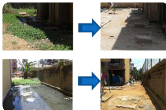
DEWATS for Lunawa Samudra Shakthi HS
