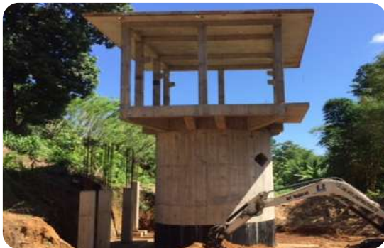
Intake Well and Pump House
