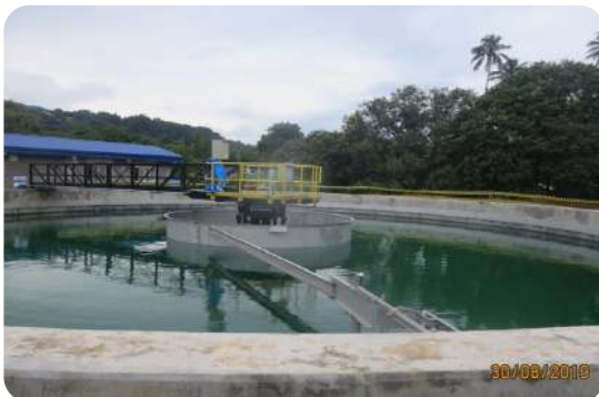
Sedimentation Tank
