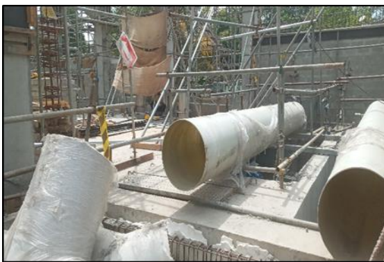
Ongoing construction at Metro Colombo Waste Water Management Project
