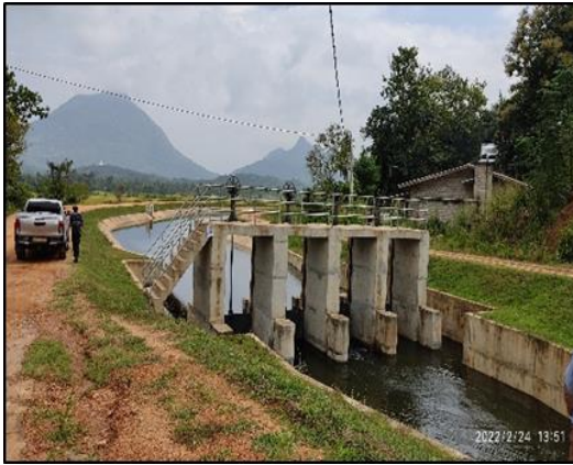
Mahaweli Water Security Investment Programme - Wemadilla Reservoir : Main Canal
