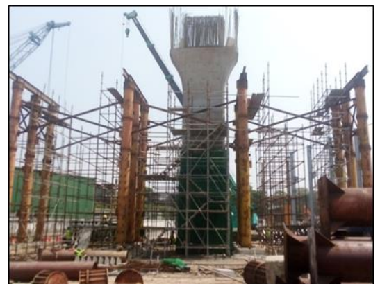
Ongoing constructions at Port Access Road
