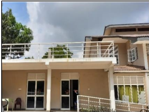
Health system Enhancement Project - Galenbindunuwewa
