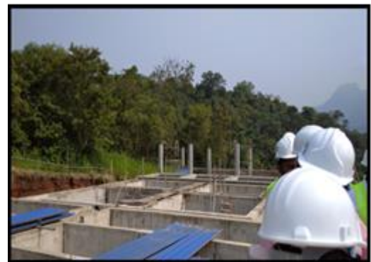
Construction of Water Treatment Plant, Wilgamuwa
