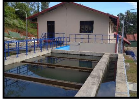
Water Supply and Sanitation Improvement Project, Galigamuwa
