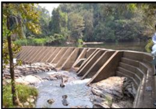
Construction of Water Intake, Wilgamuwa
