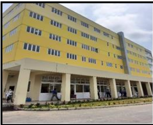
Construction of Helmouthkol Maternity Hospital, Galle
