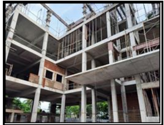
Construction of Institute Marine and Naval Study, Hapugala (University of Ruhuna)
