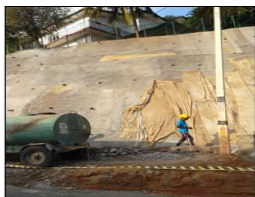
Rehabilitation of Dharmashoka Mawatha under the Kandy, Strategic City Development Project
