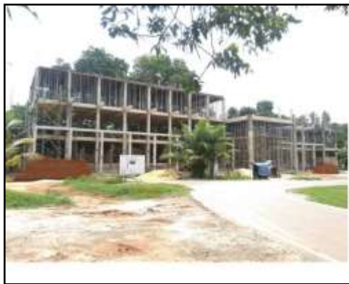
Project to Upgrading Katana, Police Academy
