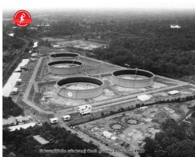
Tanks under construction in the tank farm with the process units in the background
