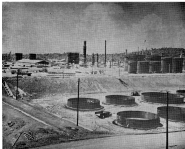
Tanks under construction in the tank farm with the process units in the background
