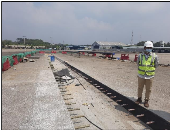
Development and Upgrading of Aviation Refueling Terminal – Bandaranayaka International Airport, Katunayaka
