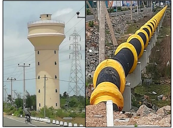
Jaffna – Kilinochchi Water Supply & Sanitation Project
