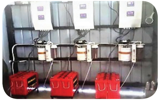
Sodium Hypochlorite generatos at Manampitiya
